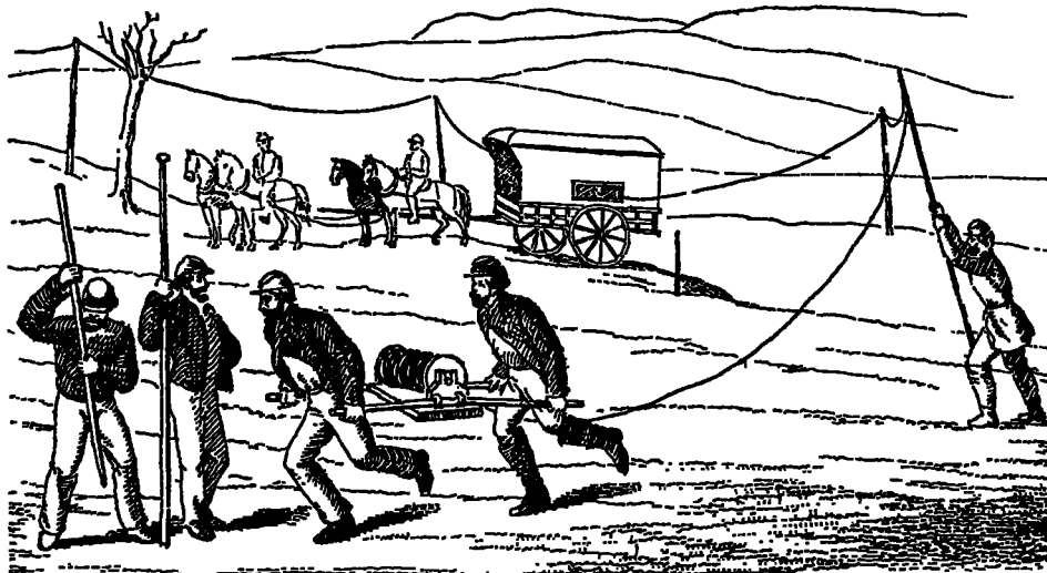
A drawing from Myer's Manual of Signals illustrating the field, or flying, telegraph. It shows the wagon with batteries and instruments. The wire (in this case presumably bare copper, since it is being strung on insulators on poles) is being run out from a reel carried by two men. The linesmen are using a crowbar to open holes to receive the lance poles. Myer estimated that 2\frac{1}{2} miles of such wire line could be put up in an hour.
